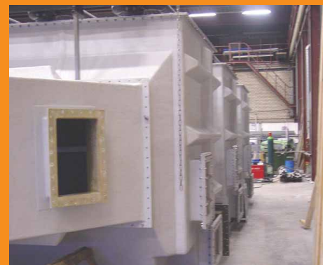
Atlac E-Nova gasscrubber in construction.
