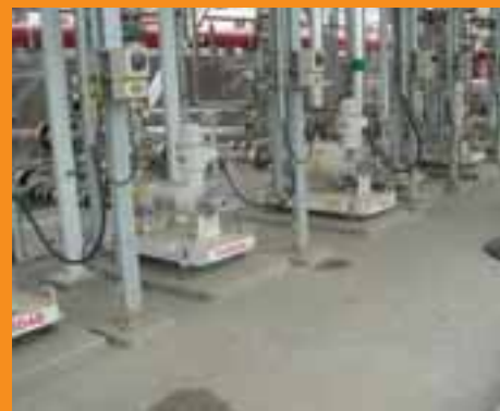
Atlac 590 floor coating at BASF in Nanjing
