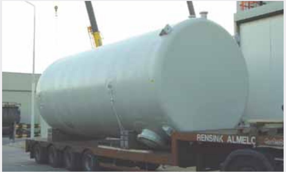
Atlac E-Nova storage tank arrives on site
