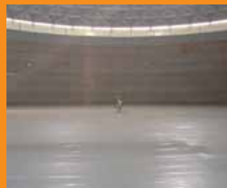
The worker indicates the size of this floating roof.
