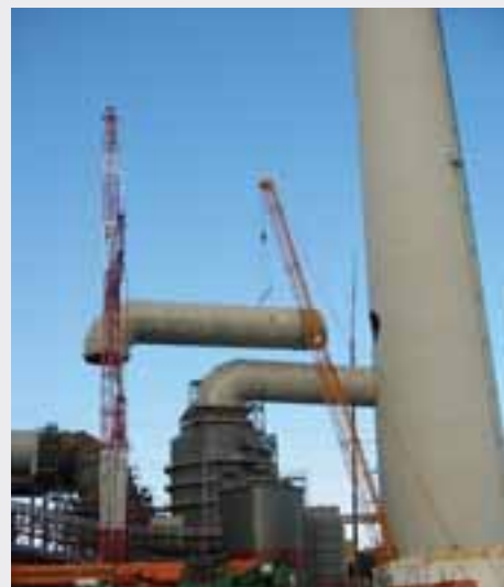
Installation on site
