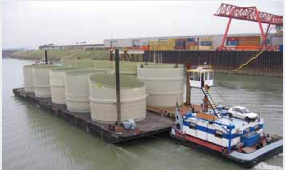
Eight meter diameter chimney sections being transported
