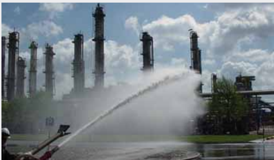
DSM Site in Geleen - fire water, a very important utility
