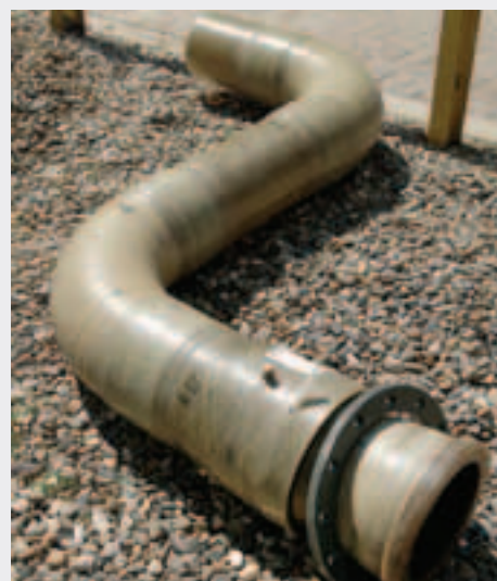
Elbow section ready for installation.
