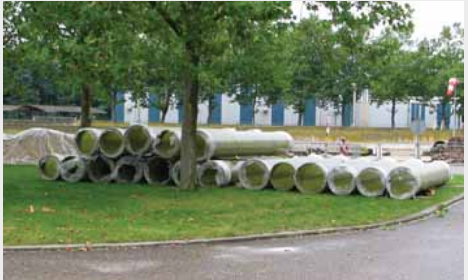
Atlac E-Nova pipes just arrived on site.
