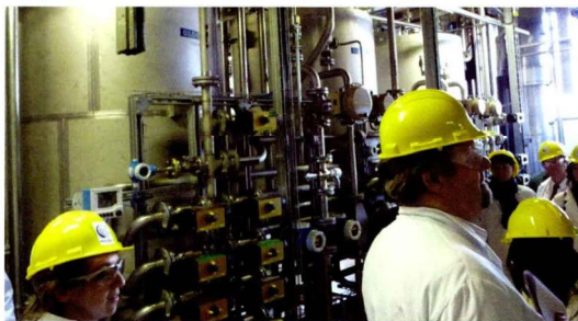
A filtration system consisting of three columns, measuring devices, process controls and computer systems was built three years ago and cost four million Swiss francs ($4.29 million).
