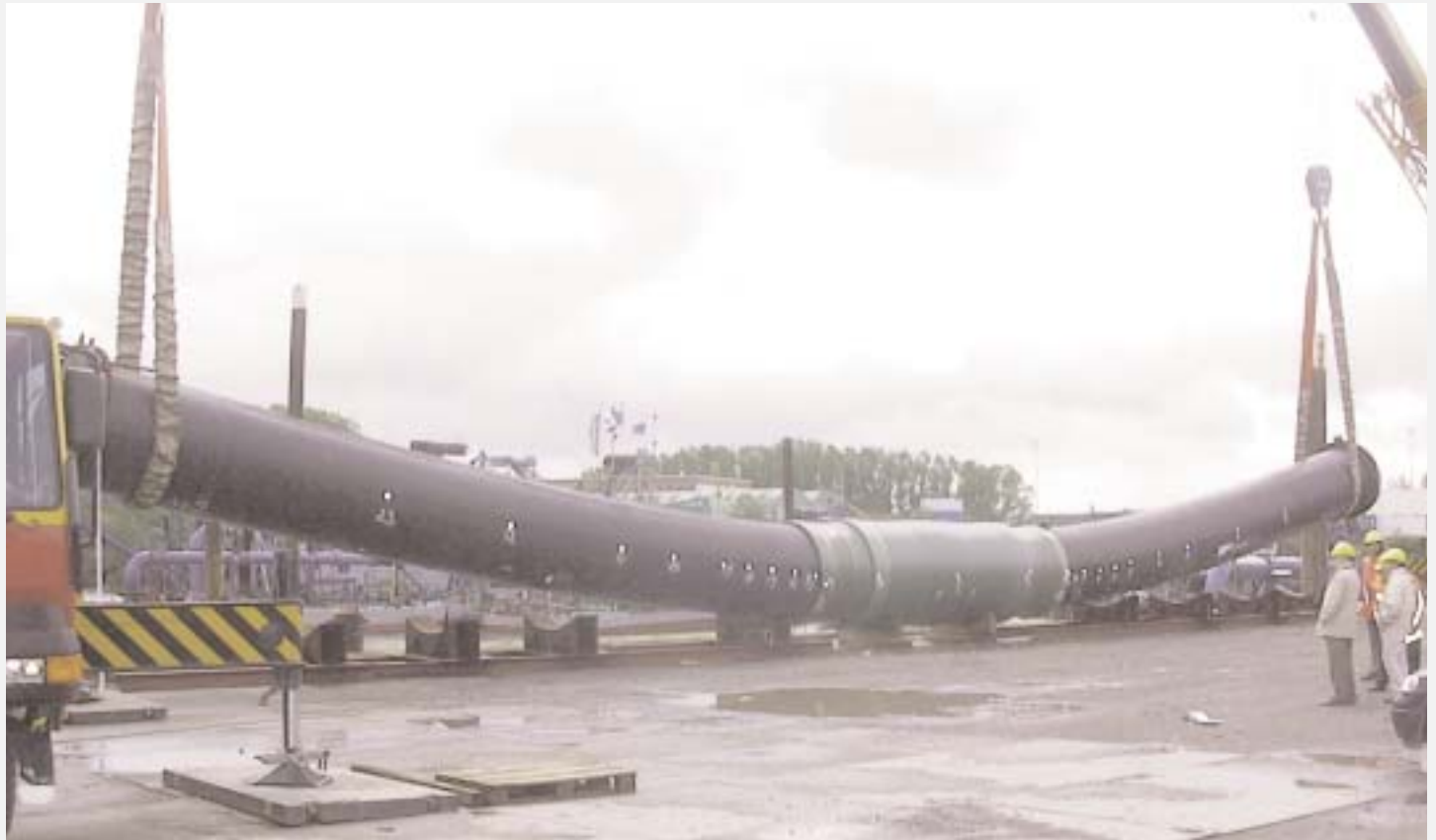
Pressure test bending of the pipe and coupling
