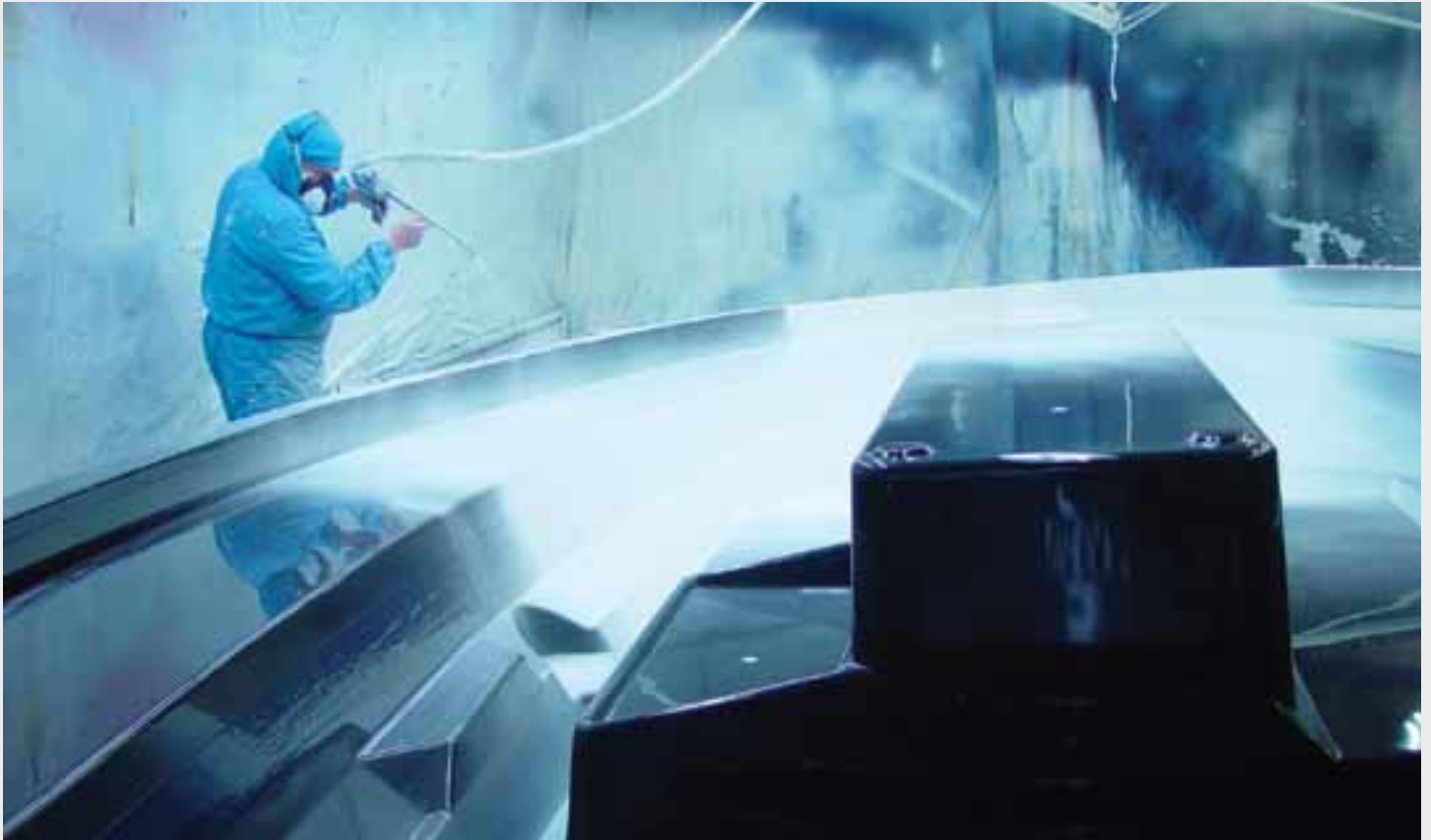
Spraying Neogel ECO onto a deck mould
