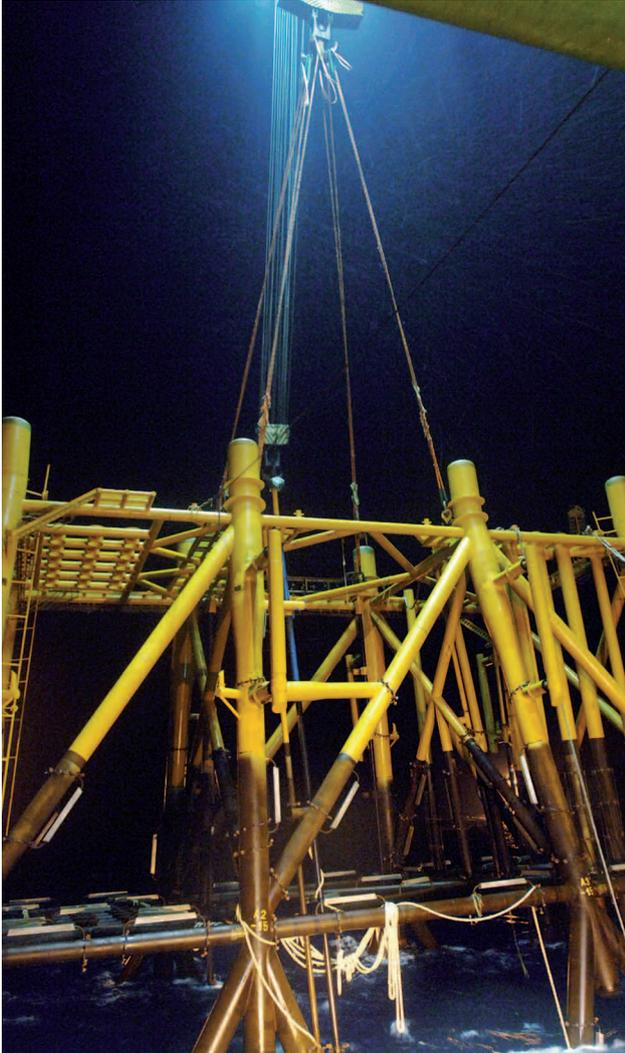
Slings made with Dyneema® also help the bottom line in other ways. They are highly resistant to abrasion as well as to exposure to UV radiation, chemicals and salt water. Lifting slings made with Dyneema® are much less likely to be compromised by the elements and can be used time after time. In short, they are made to last longer, which can greatly reduce replacement costs.
