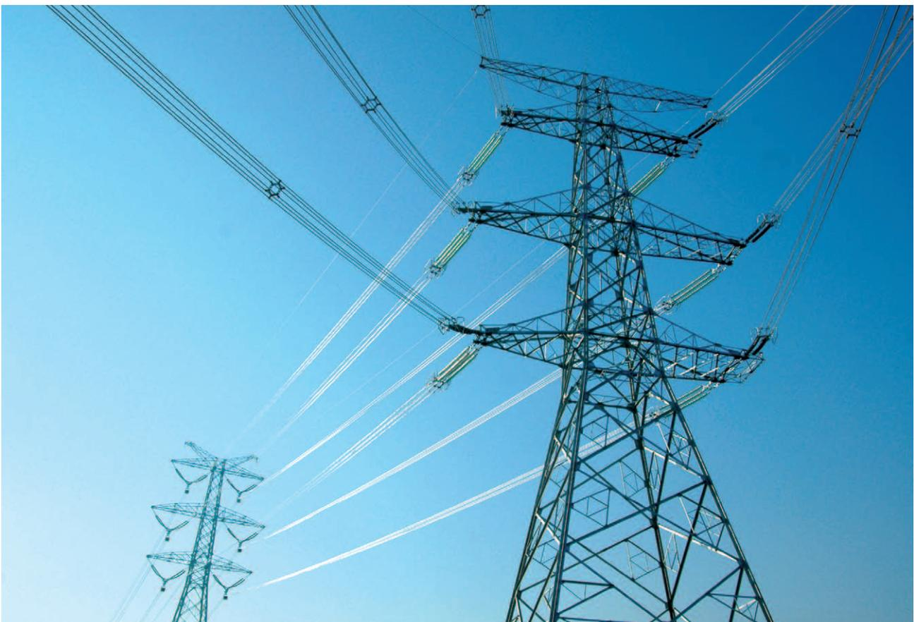
Shanghai Power was engaged in the second expansion of the Shanghai Wai Gao Qiao power plant. They needed to pull power transmission cable from the Wai Gao Qiao power plant to the Shanghai Nan Hui power transformation station. The total distance is about 40 km. The line is a 500 kV, Alternating Current (AC) grid.
