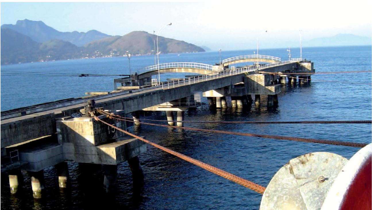
*Vessel berthed at the Angra dos Reis Terminal. Cable with Dyneema® integrated into the ship mooring, along with the steel cables.*
