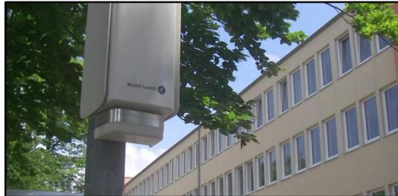
**Figure 3. A Microcell Antenna Mounted on a Pole (Courtesy of Alcatel Lucent)**
